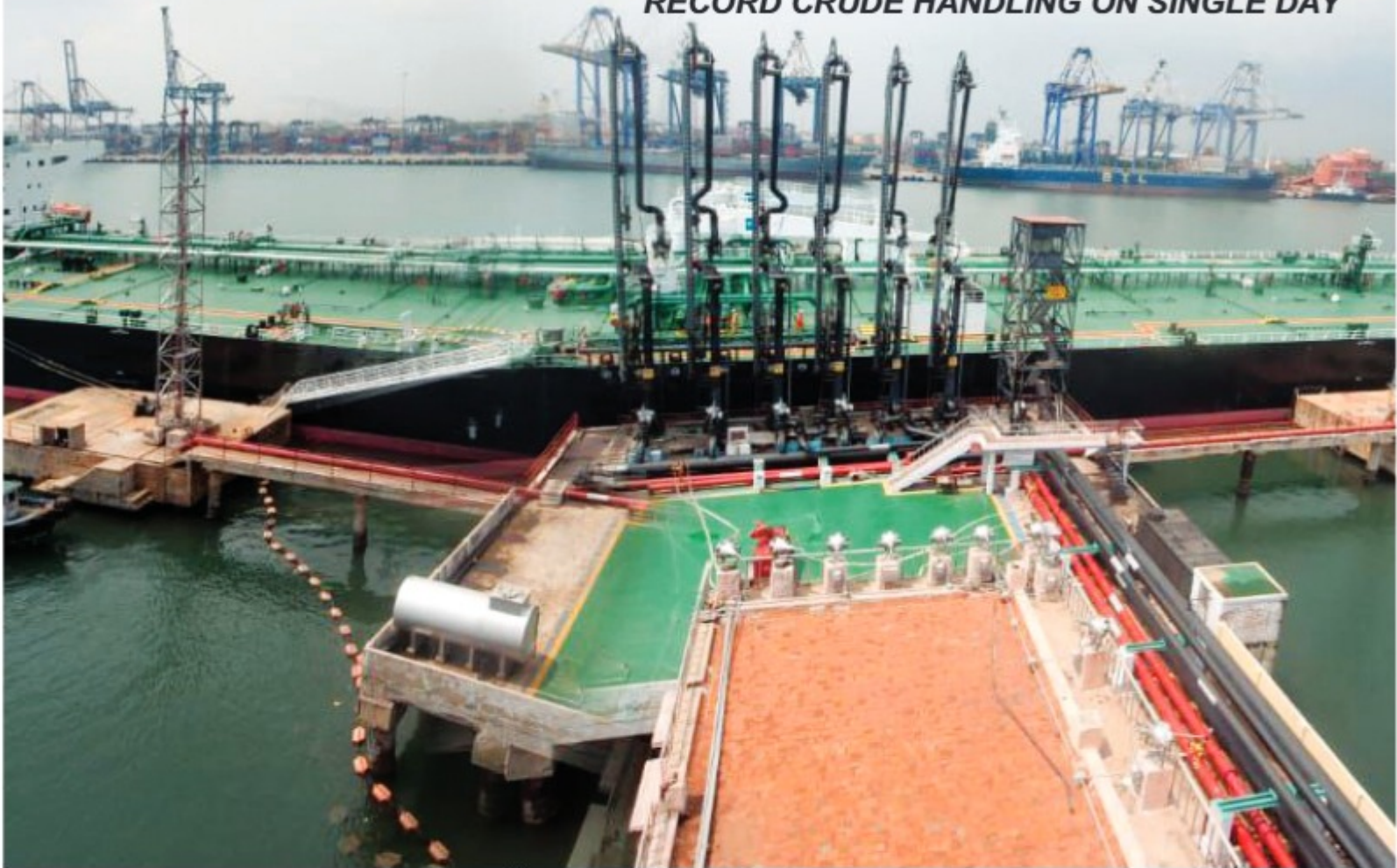
RECORD CRUDE HANDLING ON SINGLE DAY
