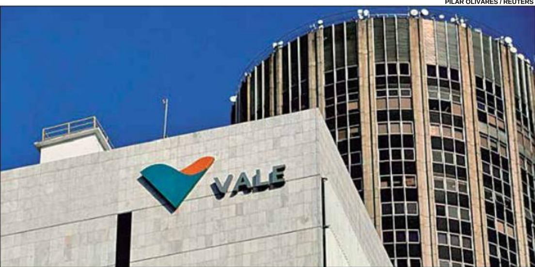
The company has operated the terminal since 2002 and the unit has the capacity to ship 25,000 t of iron ore per hour
