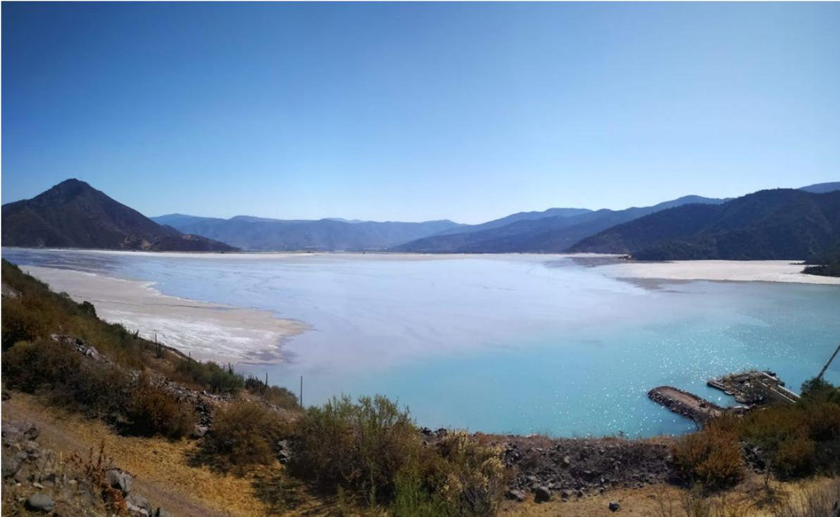
*The El Torito tailings dam at El Soldado Mine, Chile: water reclaim pond and barges, wet beach and sand wall in the distance.*
