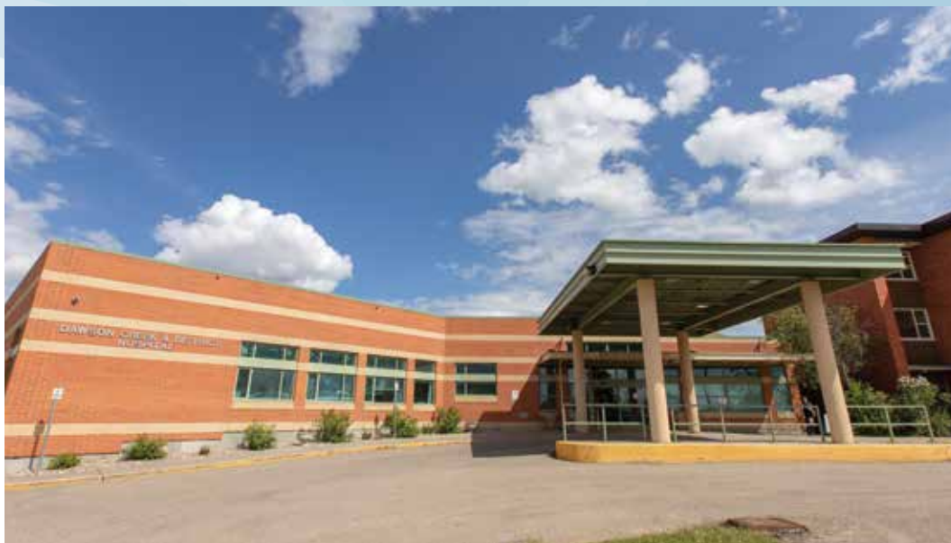
Dawson Creek and District Hospital
