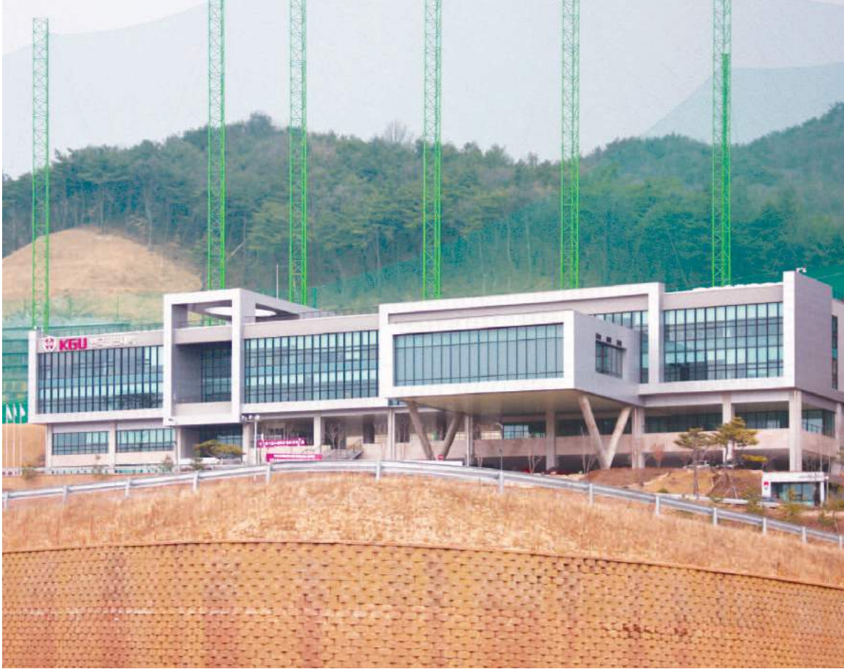
Cheongwu Golf College main building (Won the 5th Korea Civil Engineering & Architecture Award)
