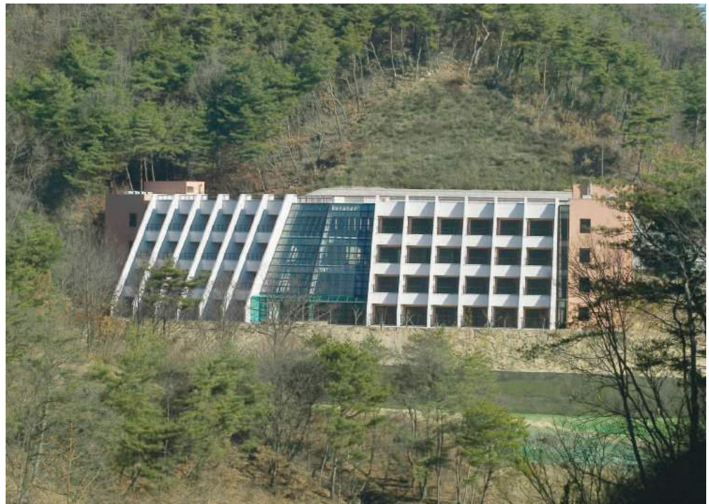
Cheongwu Golf College dormitory (Won the 5th Korea Civil Engineering & Architecture Award)
