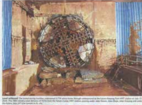
Level achieved The tunnel boring machine (TBM) cutterhead is shown in a construction site, with workers visible around it.
