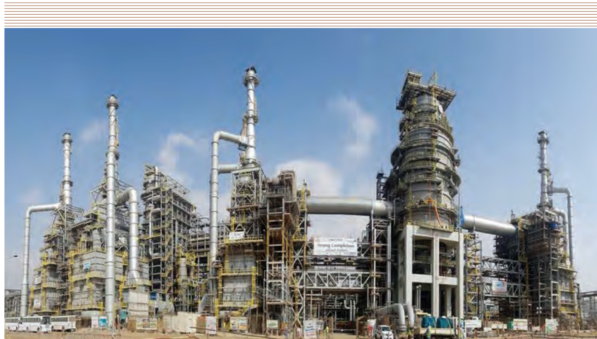
Jazan Refinery & Terminal Project
