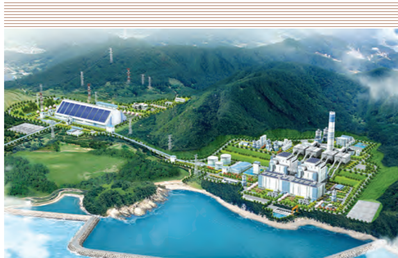
GOSEONG HAI Thermal Power Plant Project
