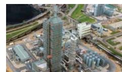
CO 2 recovery plant in the US
