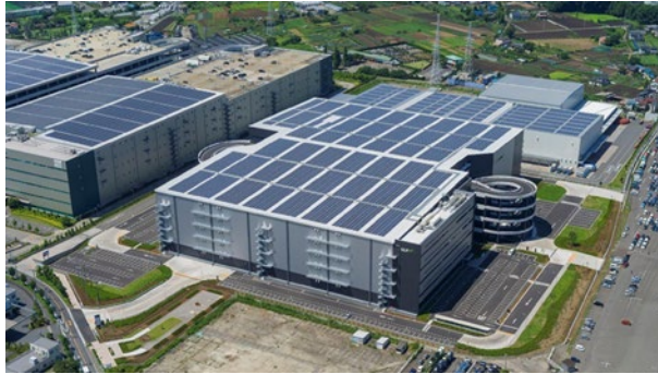
“GLP Zama” for the development of GLP Japan Inc. Total floor space: 131,762㎡ Construction in Zama City, Kanagawa Prefecture, completed in 2015
