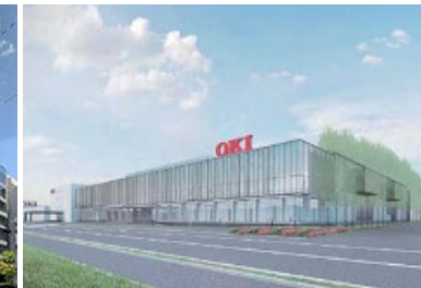
OKI Honjo Plant H1 Building (The first ZEF project completed in April 2022)
