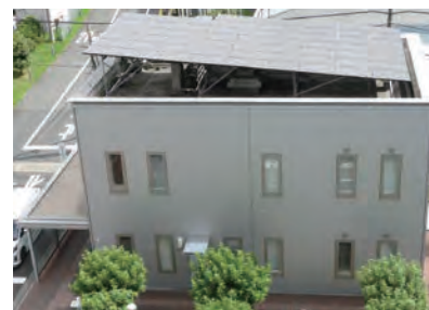
Installation of energy-saving equipment (solar power generation)
