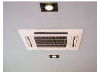
Upgrading production/air-conditioning equipment to high-efficiency models
