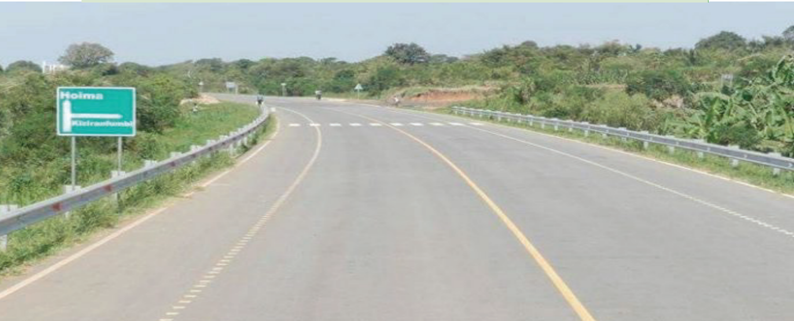
Figure 4: Hoima-Butiaba-Wanseko Road (111 Km)
