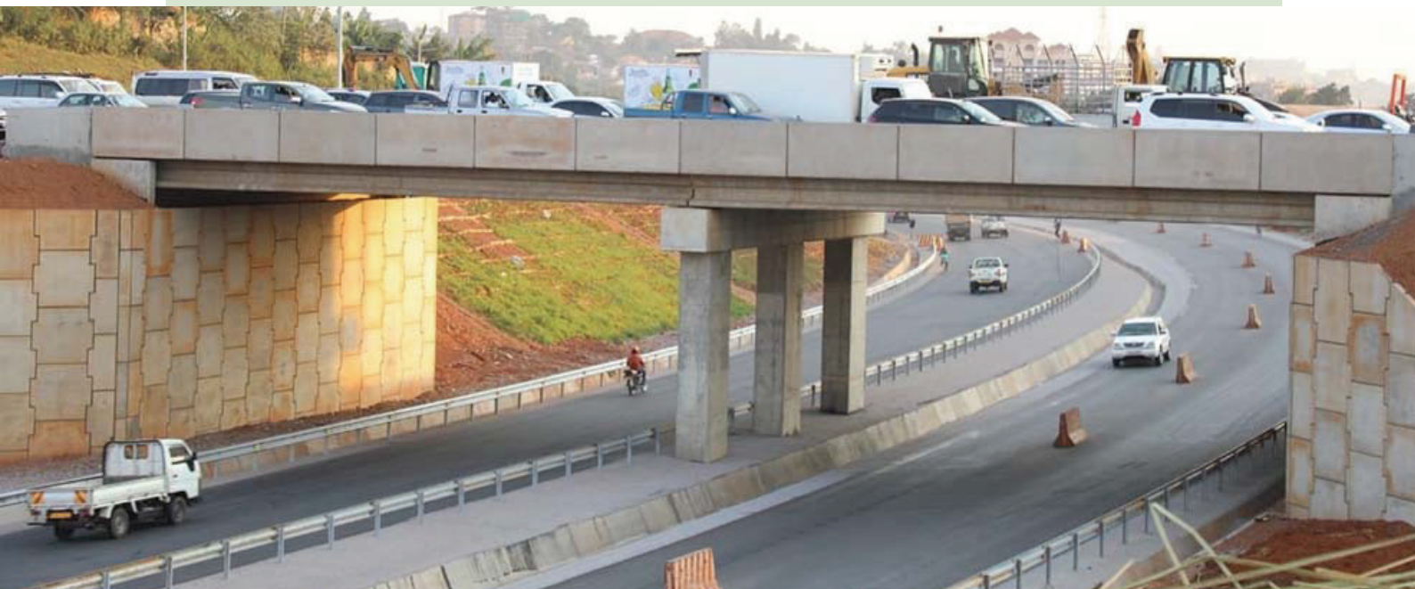
Figure 3: the Kampala Northern Bypass
