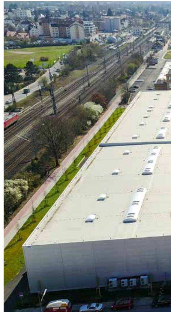
Series production facility in Langen
